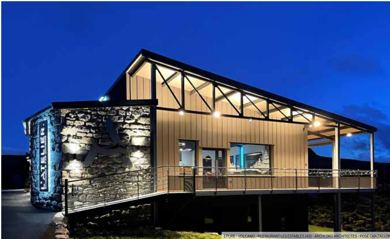
EPURE - VOLCANO - RESTAURANT LES ESTABLES (43) - ARCHI OKO ARCHITECTES - POSE CHAZALLON
