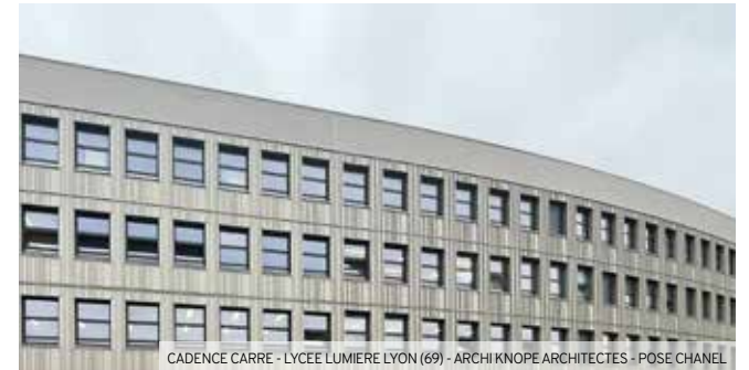
CADENCE CARRE - LYCEE LUMIERE LYON (69) - ARCHI KNOPE ARCHITECTES - POSE CHANEL
