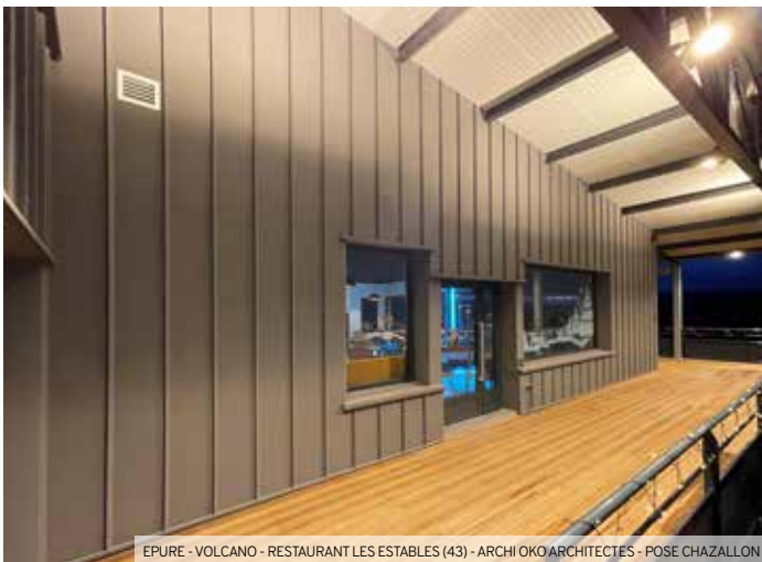
EPURE - VOLCANO - RESTAURANT LES ESTABLES (43) - ARCHI OKO ARCHITECTES - POSE CHAZALLON
