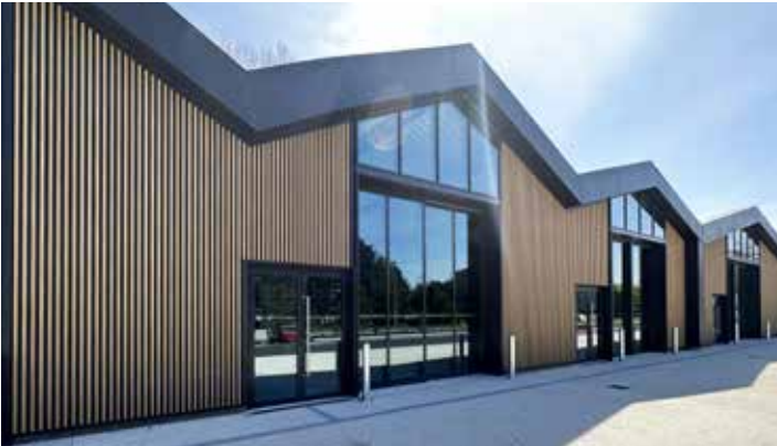
ON WOOD BARO 710 - -NATURAL OAK - BATIMENT - FENOUILLET (31) - ARCHI HOYER ARCHITECTE - INSTALLATION LABEDAN
